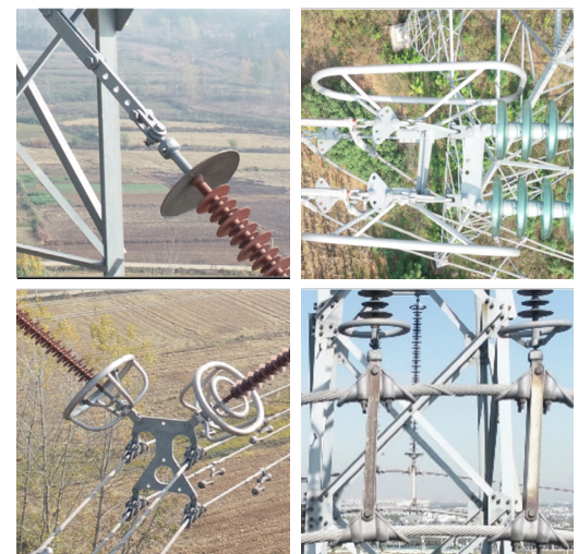
Detailed Inspection Views
